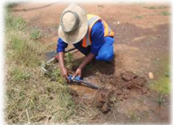
Repairing leaks will reduce physical losses
