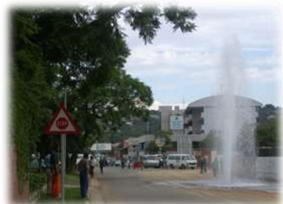
Burst pipes contribute to physical losses
