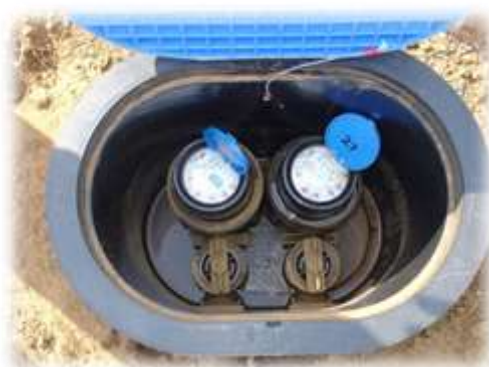
Double meter box considered as two connections
